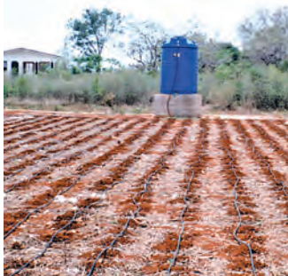
Gravity drip irrigation system
