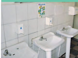
Hand-washing stations/facilities should exist in the same ratio as toilets. Soap, single-use towels and potable drinking water should also be provided.
